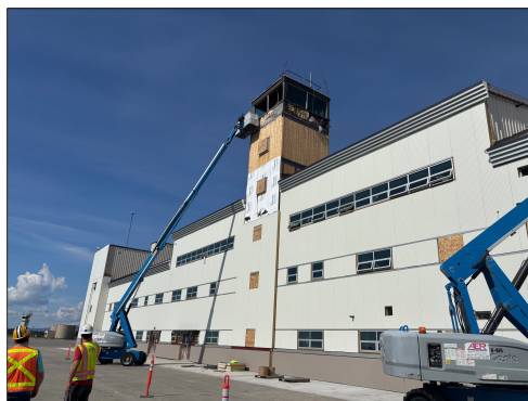
Building 1557 Thermal Envelope repairs at Ft. Wainwright, Alaska.
