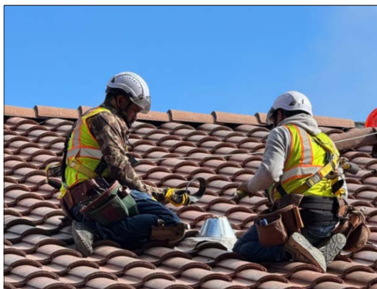
Roof replacement project in Presidio of Monterey, California.
