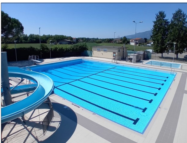
Swimming pool and pumphouse renovation at Aviano Air Base, Italy.
